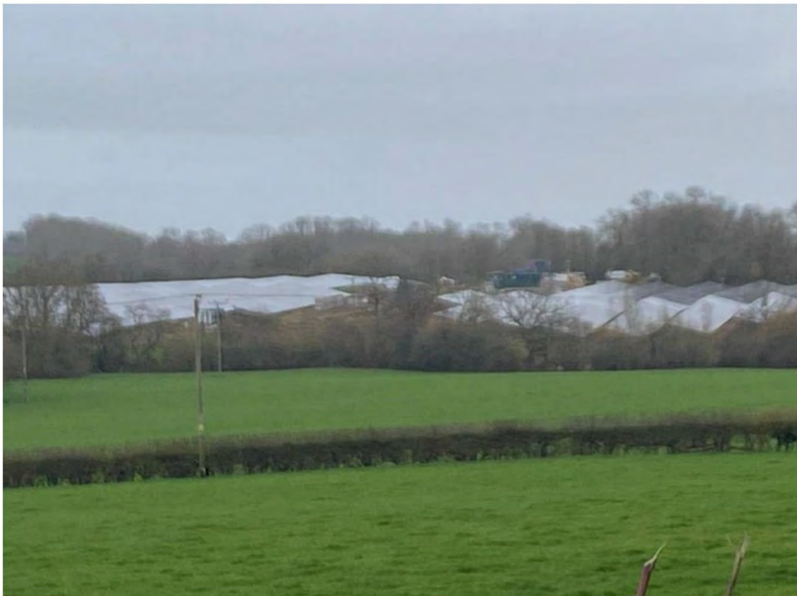
VIEWS TODAY SOLAR PANELS 3M HIGH
